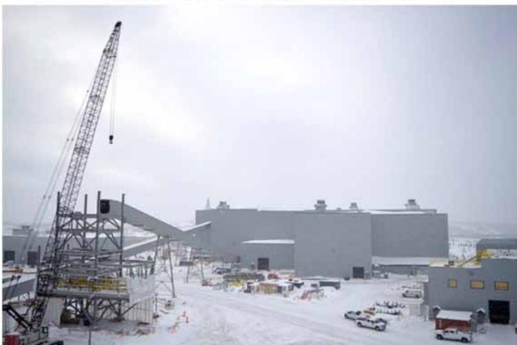
Exhibit 1: Renard Mine Site - mill construction progressing
