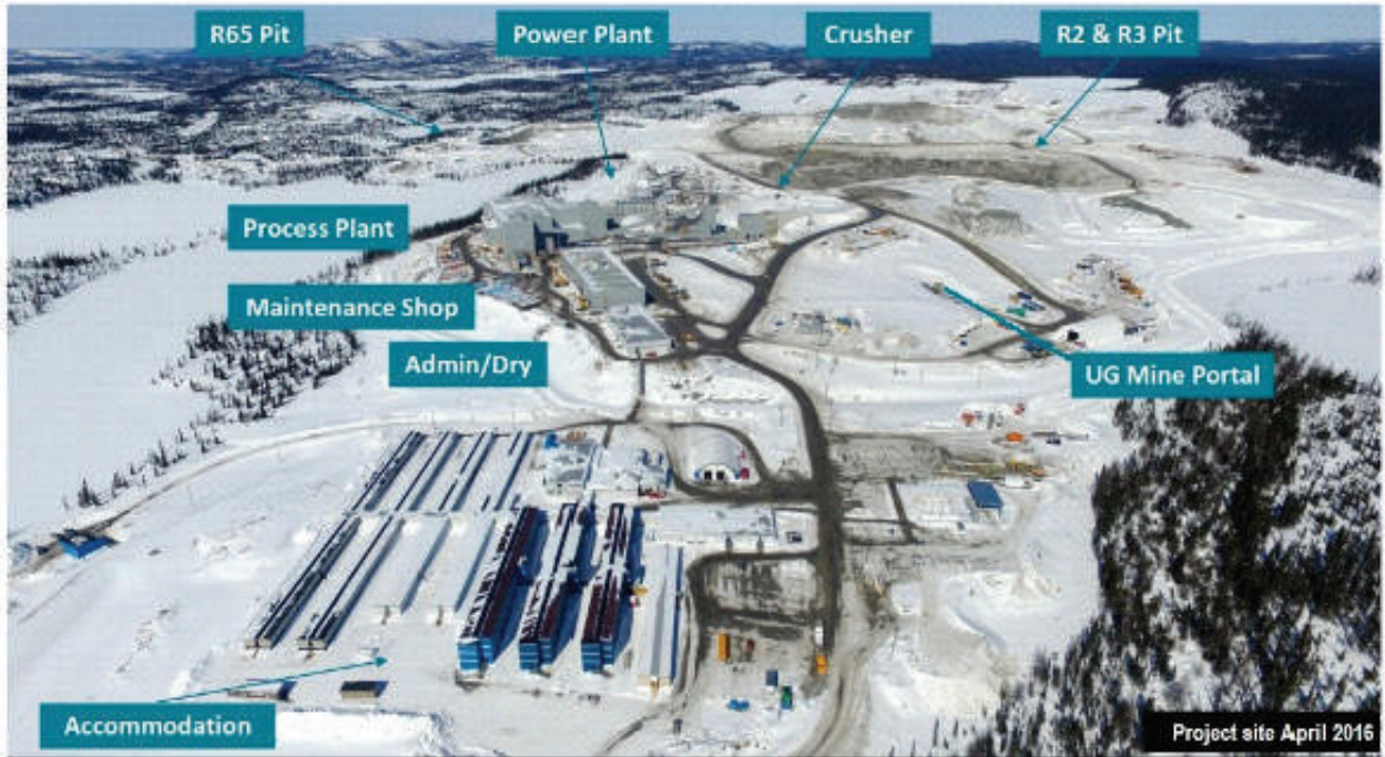
Exhibit 1: Renard Mine Site - Construction progressing very well
